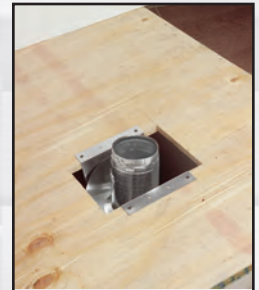
Push pipe through vent support.
